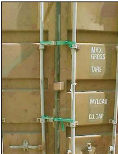
Doors secured using correct strap and buckle.
