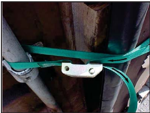
Correct threading of strap through buckle.
